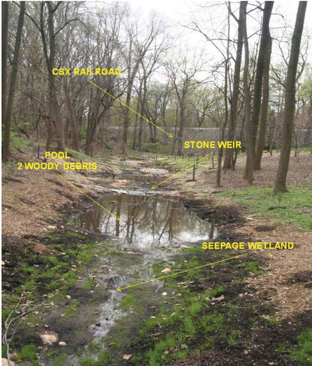
Location C : Post Construction Left Tributary Facing Upstream
