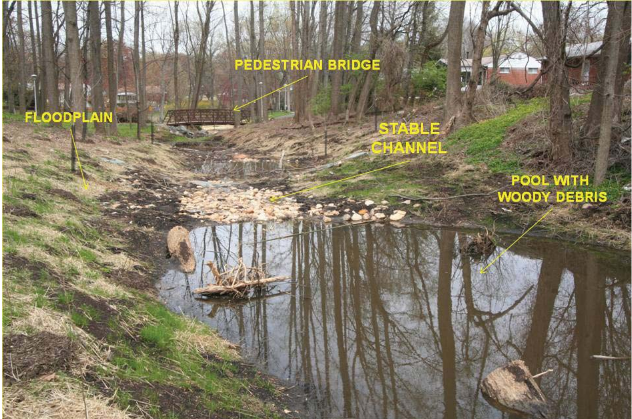
Location B: Post Construction Left Tributary Facing Downstream at Wetland
