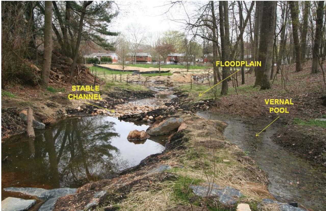
Location A : Post Construction Right Tributary Facing Downstream
