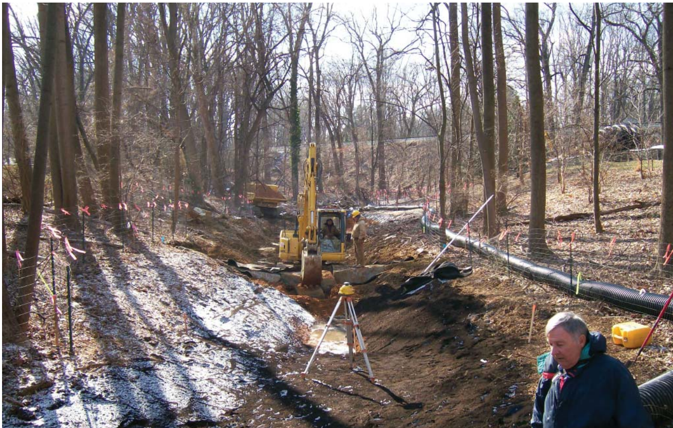
Location A: Stepped Pools under Construction Facing Upstream
