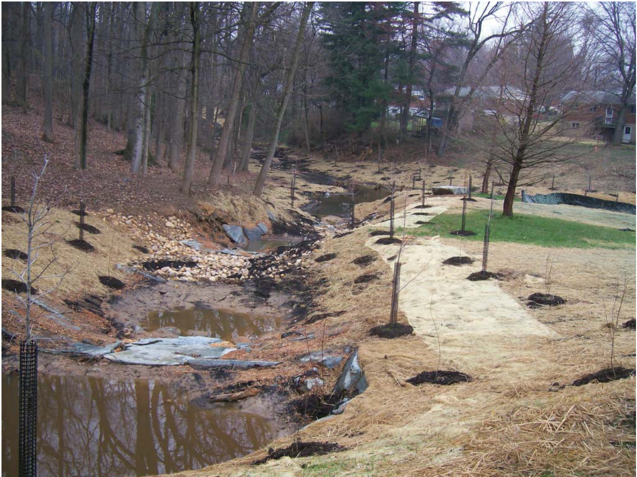
Location A: Completed Stepped Pools Facing Upstream
