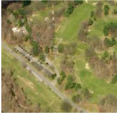
Existing Facilities Aerial
